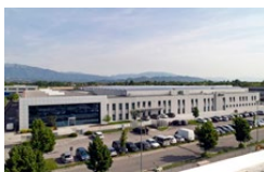
Photo 3: Steelco plant in Riese Pio X Photo: Steelco
